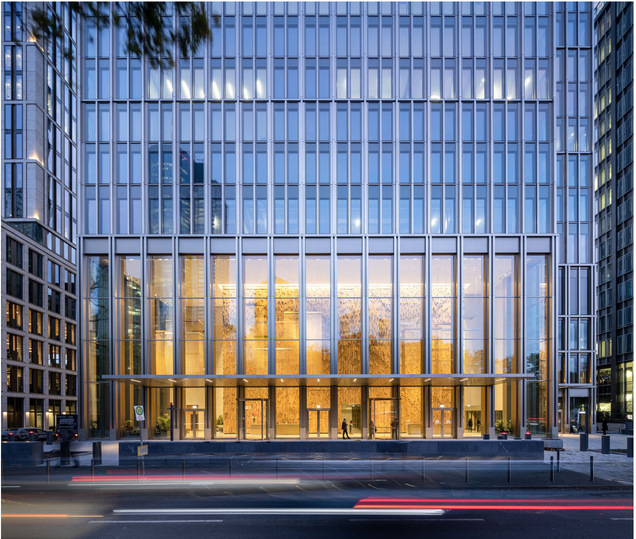
Figure 3: The concise, vertically structured window facade made of glass and anodized aluminium of the four-story high entrance area was implemented with a mullion-transom facade from the HUECK Trigon 60 series. (source: ©Pecan Development)
