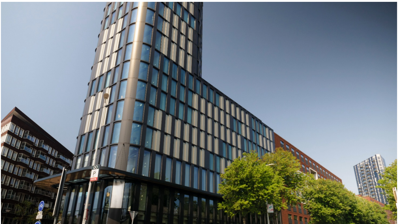
Figure 1: An essential part of the energy and sustainability concept is the “living” façade made of glass and aluminium. Following careful testing, aluminium proved to be the most sustainable material in this context. (Source: HUECK)
