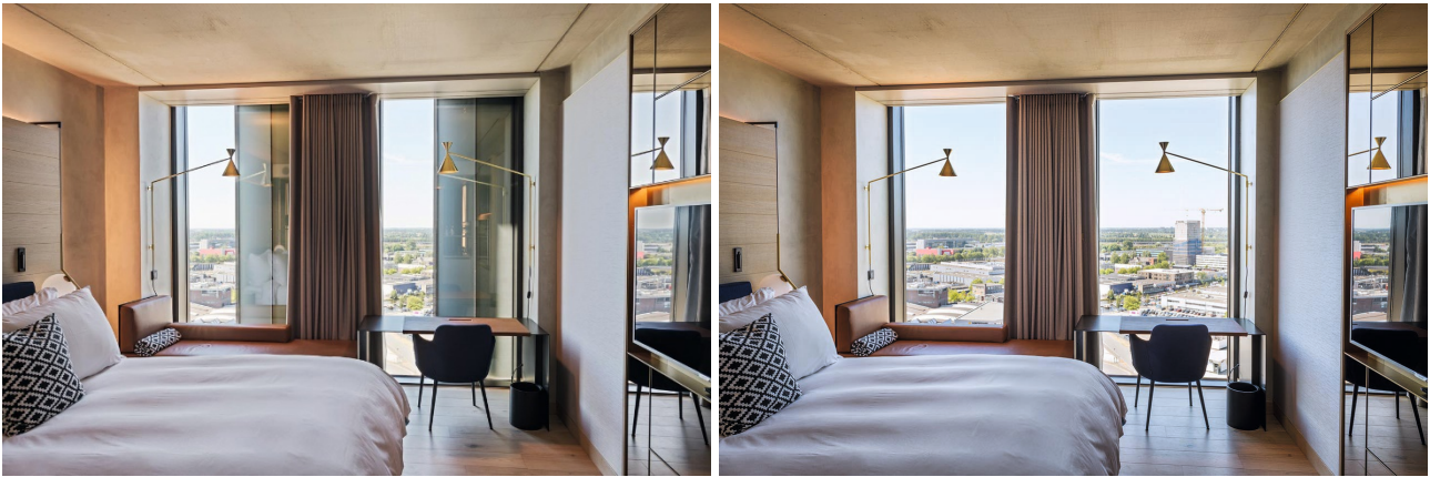
Figures 3 and 4: While the guest is not in the room, the sliding elements in front of the storey-height glazing are closed or opened automatically depending on weather conditions. (Source: HUECK)
